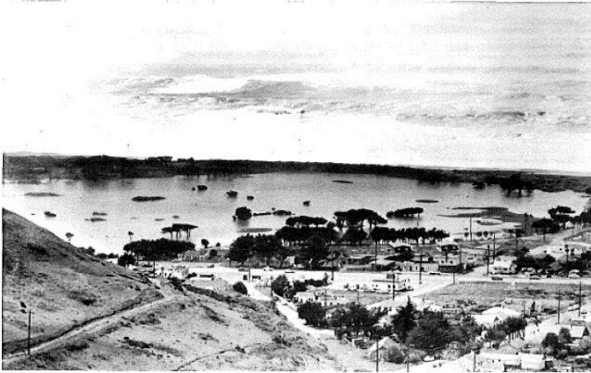
Figure 1 April 4, 1958 flooding of Sharp Park. Caused by storm water runoff and wave overtopping of berm. Geomatrix Consultants. Feasibility Study, Restoration of Coastal Embankment, Sharp Park Golf Course, Pacifica, California. November 1987. p. 20.
