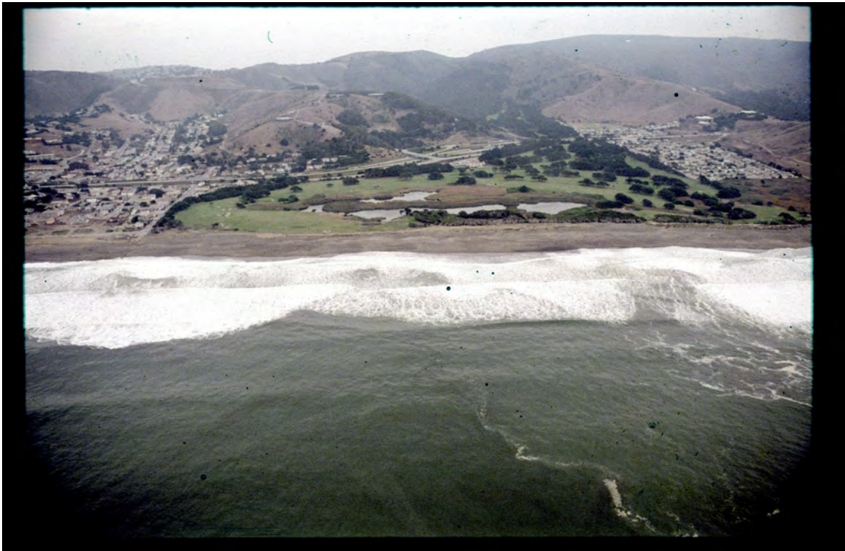
Figure 4 1979 Coastal Records Project photo showing incomplete berm at Sharp Park.
