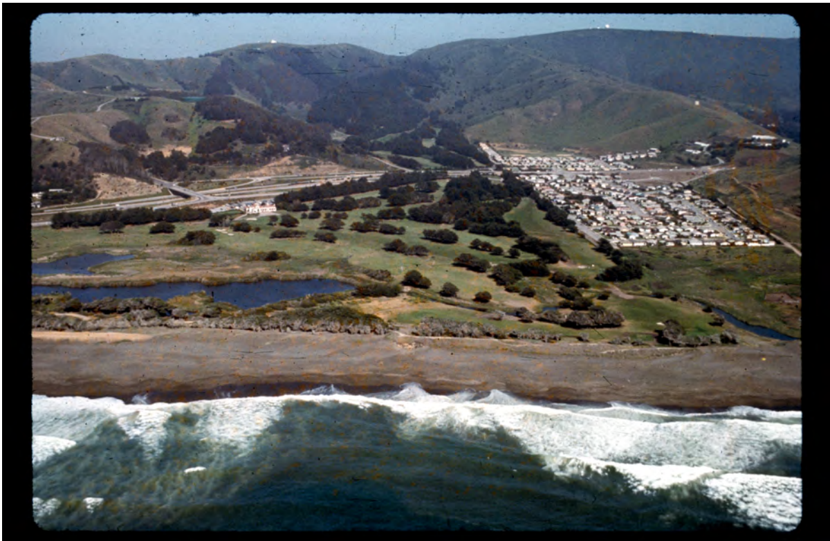
Figure 3. 1972 Coastal Records Project photo showing incomplete berm at Sharp Park.
