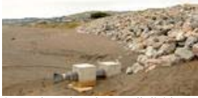
An earth-and-rock seawall divides the Pacifica shoreline from Sharp Park Golf Course.
