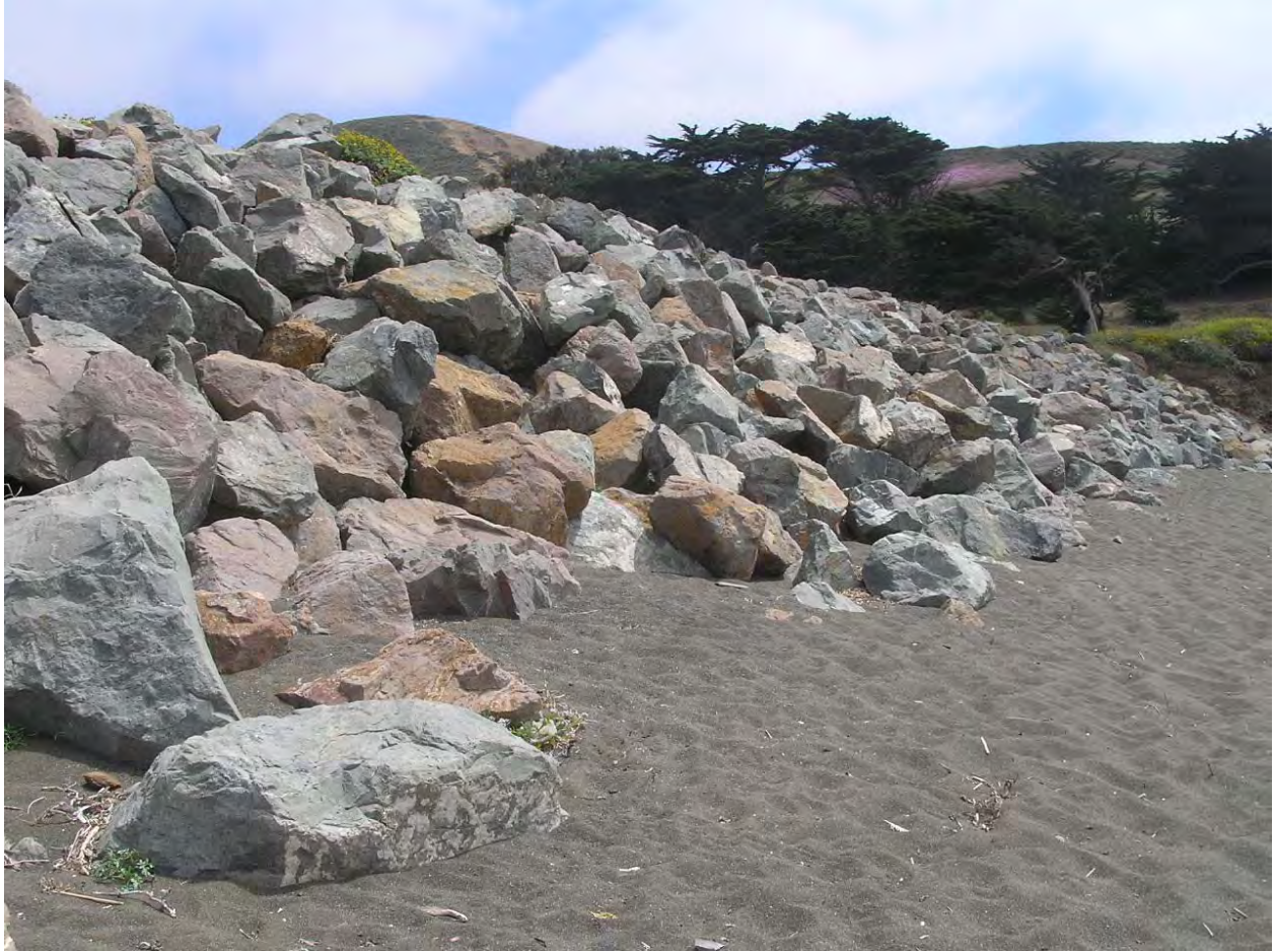
Figure 14. Beach armoring (boulder revetment). The historic location of the lagoon outlet, near the modern pump outfall, is completely armored by an engineered boulder revetment approximately 3 m above the adjacent beach. The seawall and revetment preclude natural lagoon outlet from forming and draining impounded floodwaters in Laguna Salada by gravity following natural breaches.
