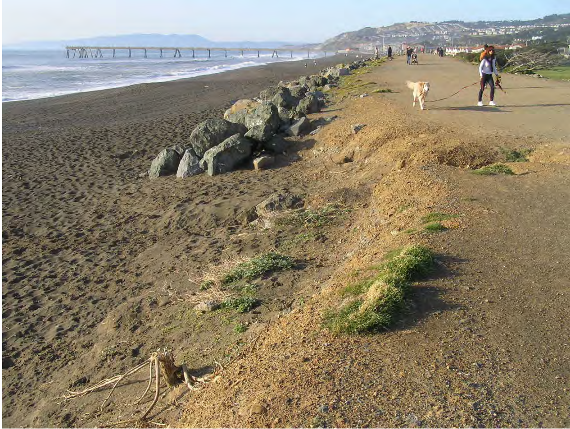
Figure 13. Armored and earthen “seawall” profiles. Erosional scarp in earthen berm “seawall” at south end of boulder armoring. No eolian (wind-deposited) dune sand occurs within or in lee of boulders, or on landward slope of berm. Adjacent beach is coarse sand. Small patches of native dune vegetation (beach-bur, Ambrosia chamissonis ) occur at the toe of the scarp or boulders.
